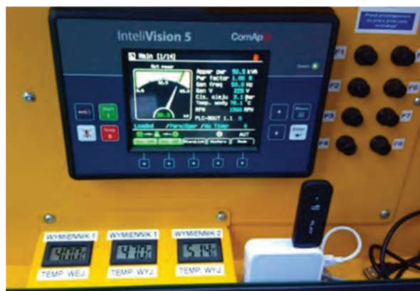
Fig. 5. Control panel during parameters reading. In the center, the main ComAp controller, below current water temperature readings at the heat exchangers. At the right – remote control module.
