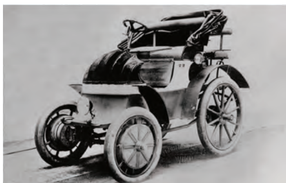
Fig. 1. The in-wheel motors vehicle developed by Lohner and Porsche in 1898 [10]
