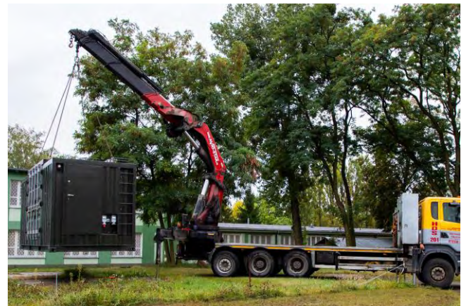
Fig. 9. The diag- dyno station during unloading using a hydraulic truck crane
