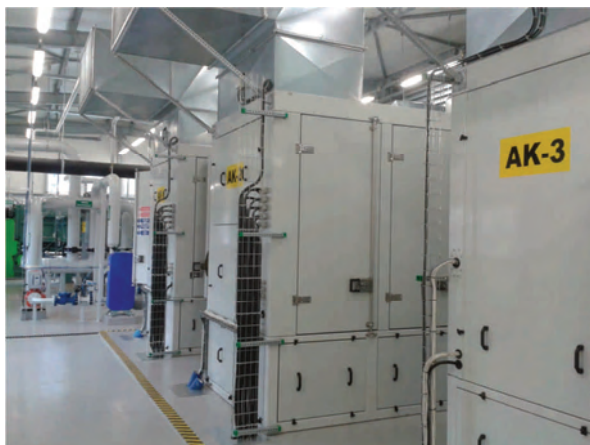
Fig. 6. Power generators with electronically controlled, post-processing gas injection system, located in one of the "AZOTY S.A." plants
