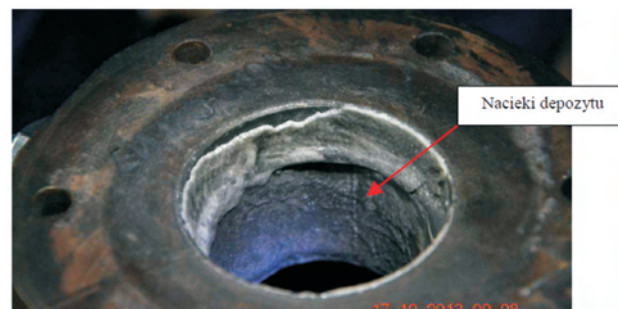
Fig. 13. Internal wall after the tests with cooled exhaust pipe (entry to the pipe) [7]
