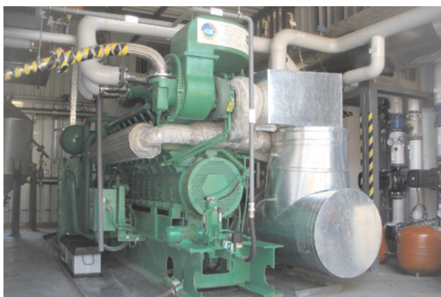
Fig. 1. The biogas cogeneration set with the GE JENBACHER JMS 316 GS-B.LC engine operated at the WARTA S.A. Sewage Treatment Plant of Czestochowa
