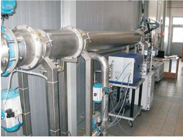
Fig. 4. Dilution tunnel downstream view, showing System 1 connected to the dilution tunnel
