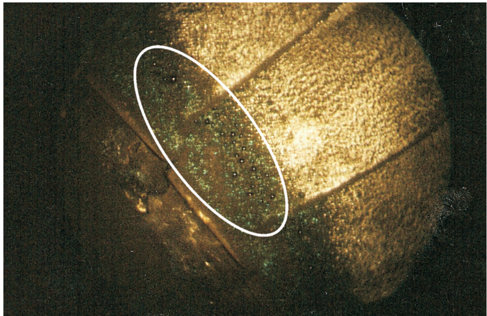
Fig. 5. Characteristic high temperature corrosion bubbles on the guide vanes of the high pressure turbine of the Zorya DE59 engine
