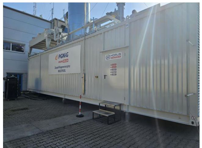
Fig. 6. The containerised cogeneration unit with the Perkins 4016-61TRS2 industrial gas engine at Horus-Energia industrial engines test facility
