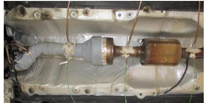
Fig. 5. Prototype SCR system installed with measuring equipment
