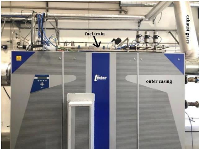
Fig. 10. Turbec T100 PH microturbine system [5]
